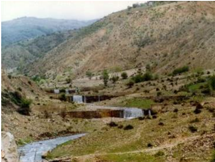
Figure 28: Check dams in the Kamenicka river bed (system of check dams in the river bed)
