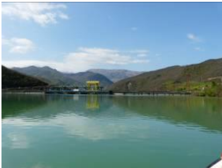
Figure 7: The UHPP dam and its lake
